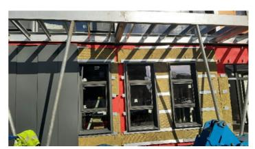
Three simple shrouds manufactured for the demonstrator building
